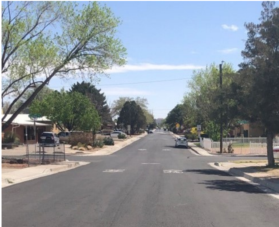
Figure 5: Alvarado Drive Looking South
